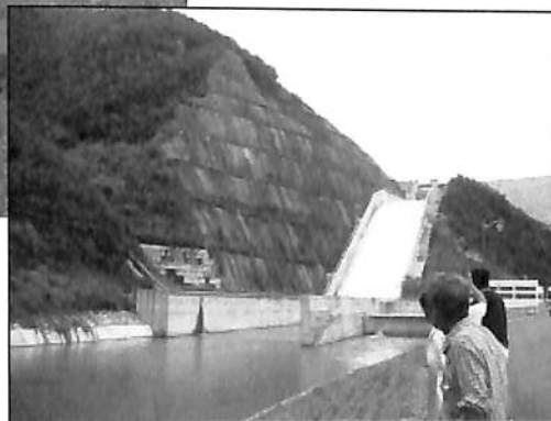
Grass seeding on the cutting face(Donghwa dam)
