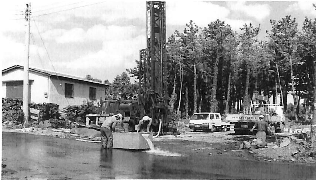
Figure 7 Groundwater exploitation and pumping test
