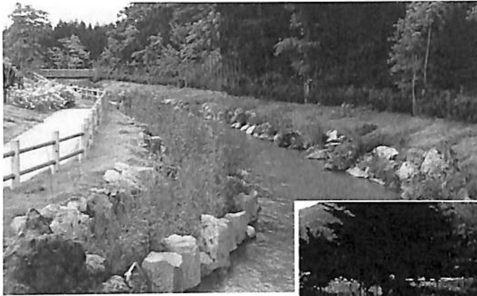
Walk way near drainage channel
