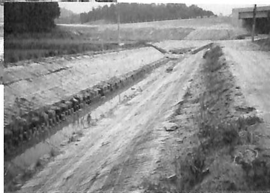
Geo-green cell in drainage channel
