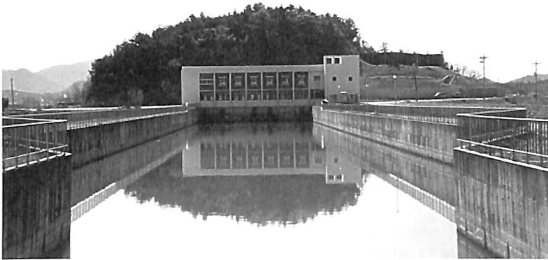
Figure 5 Goheung pumping station
