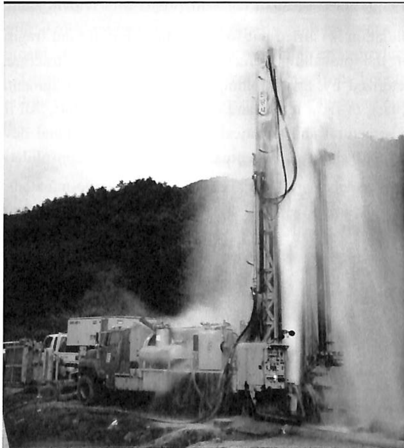
Figure 9 Drilling of tube well for groundwater exploitation
