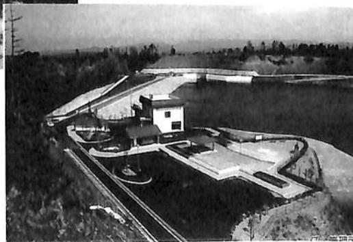
Platform for observation near reservoir
