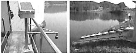
b) Intake tower
