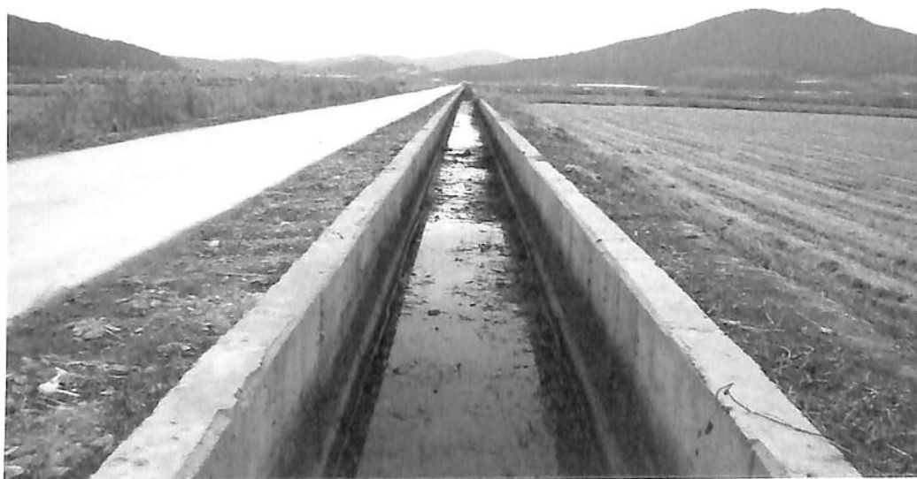
Figure 8 Irrigation canal made of concrete flume
